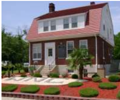
Superintendent's lodge at Wilmington National Cemetery.
