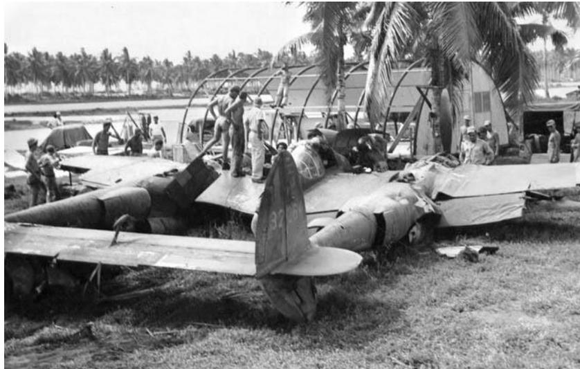
**Ground crewmen at Henderson Field inspect the damage to the P-38 that Barber flew on the mission, which sustained 100 bullet holes.**
